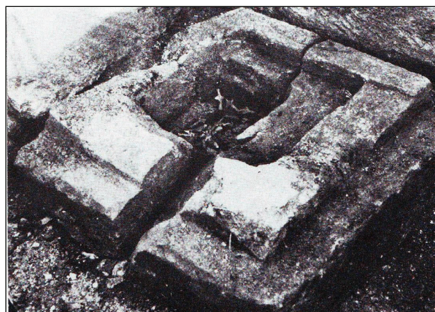
Fig. 2. The poros base-repository of the cult statue of the temple of Athena Nike during the restoration works conducted at the temple of Athena Nike from October 1935 to March 1939 by Nikolaos Balanos.
